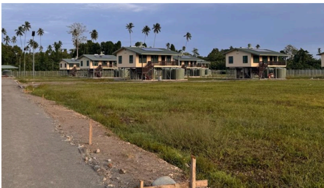
Figure 3: Enabling infrastructure under construction at the Soraken site, including staff housing units fitted with solar power and water storage.
