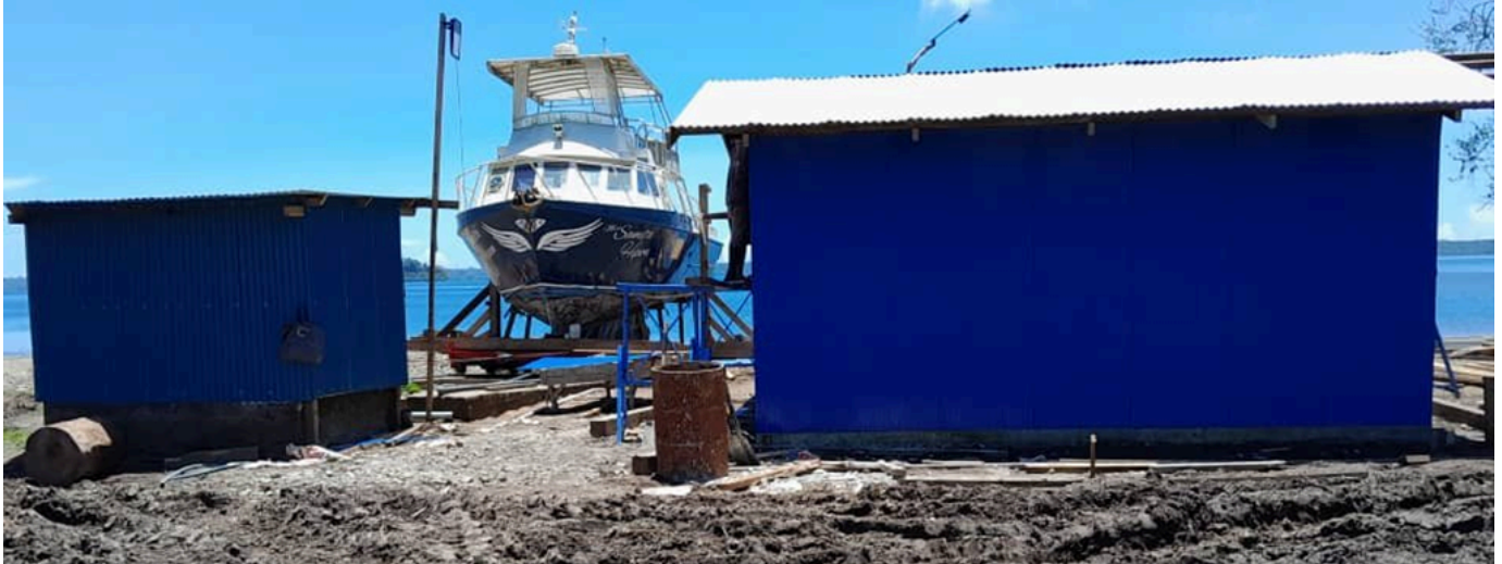
Figure 6: Existing boat-maintenance shed and slipway on the Soraken shoreline, part of the site's existing maritime and wharf infrastructure..
